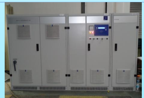
800V / 600A, 250 kW Pack Level Test System
